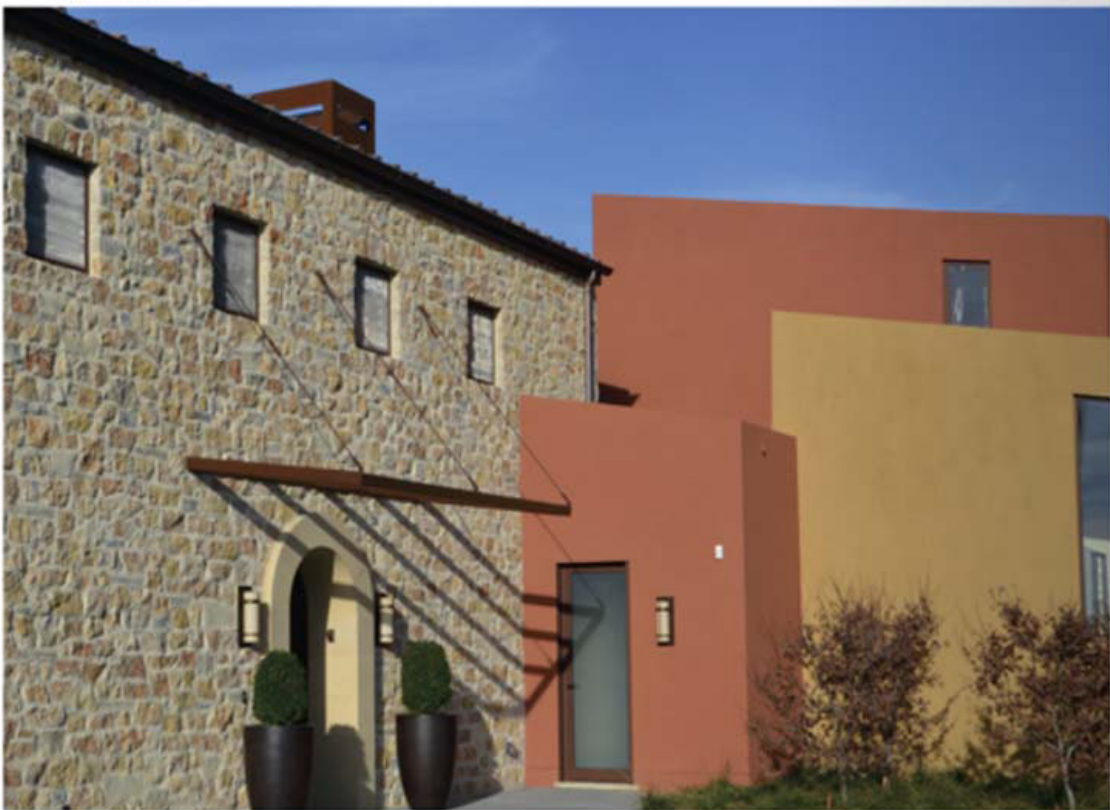
The stone walls, created of five types of stone, provide a striking contrast with the modern lines and washed earth-tone walls of the adjoining wings.
